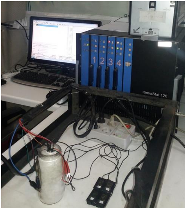
Figure 2. Battery setup and battery analyzer device
